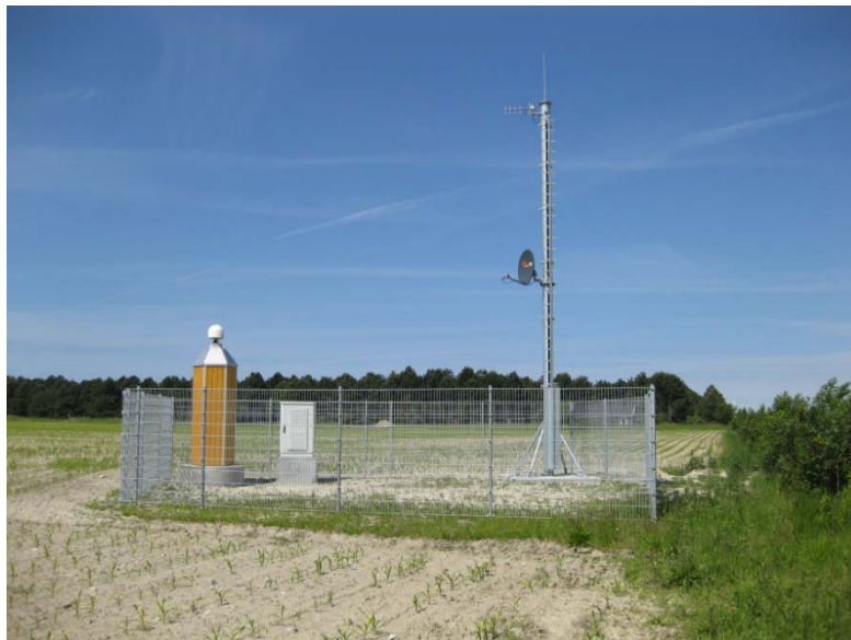
Permanent GNSS station of Femern A/S near the coast of the Fehmarnbelt. Antenna mast for data communication is located directly north of the GNSS pillar. Photo: A. Jensen.
