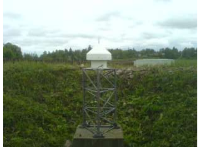
Figure IV-4. Antenna site at the EGNOS RIMS station in Virolahti. (Photo: Tomi Tenhunen)
