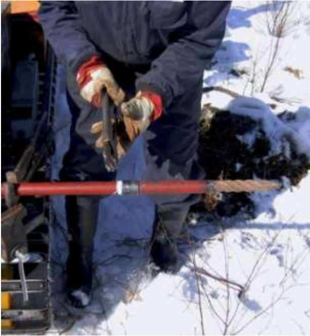
Figure II-7. Installation of the groundwater access tubes in 2009. Note the very short perforated section at this site, designed for the thin layer of ground moraine below silt and clay. (Photo: Jaakko Mäkinen)
