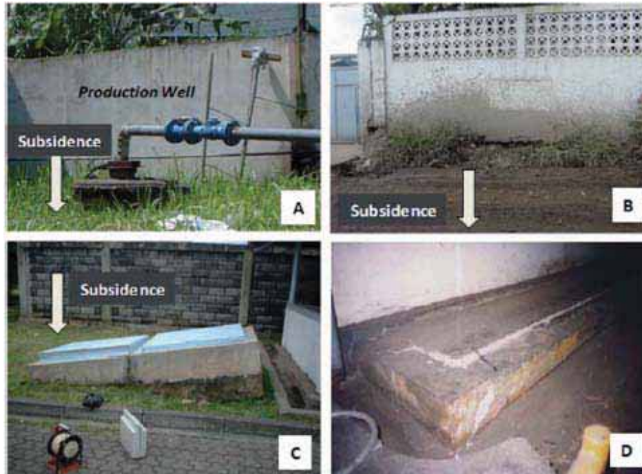
Figure 10. Examples of subsidence features in the field. A and B: ground lowering and hanging wall in the Leuwigajah area (around CMHI GPS station); C: differential subsidence around GDBG GPS station; D: structural cracking around DYHK GPS station.
