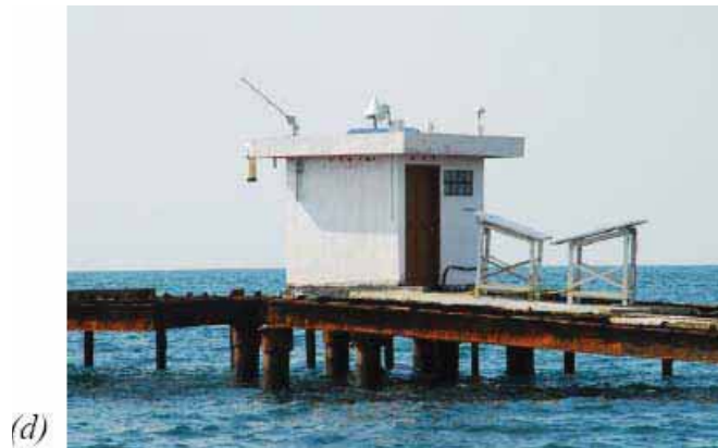
Figure 2. The IPGSN geodetic monument types: (a) on the top of concrete roof, (b) concrete pillar, (c) stainless-steel rod, and (d) on a tide gauge station. Photos are taken by Cecep Subarya.
