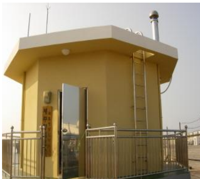
Figure 4.12 CJUN TG station with GPS antenna.
