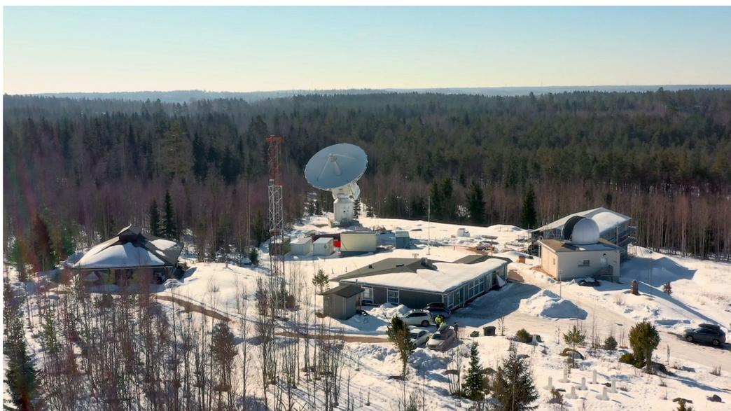
Metsähovi Geodetic Research Station. The gravimetric laboratory is at the left, the new VGOS radio telescope in the centre and the SLR observatory at the right. Behind it is the new main building.
