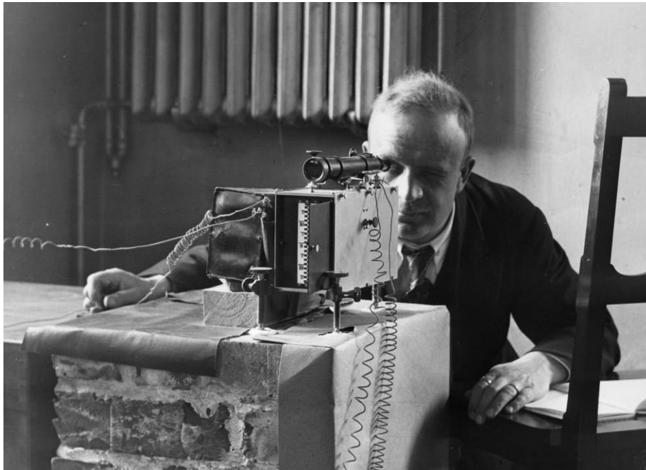
Dr Uno Pesonen observing gravity with a pendulum instrument in 1924. (Photo: FGI archives)
